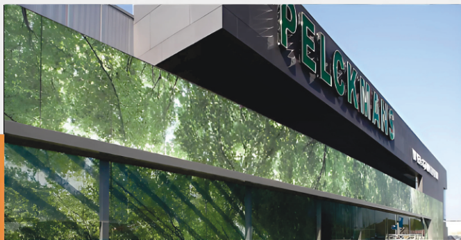
TUINCENTRUM PELCKMANS TURNHOUT, BELGIUM ARCH. BART JANSSENS
